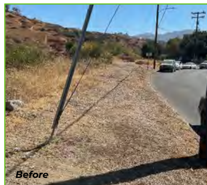
Created a decomposed granite pathway from Race Street to the Newhall Community entrance ( Make a Difference Day )
